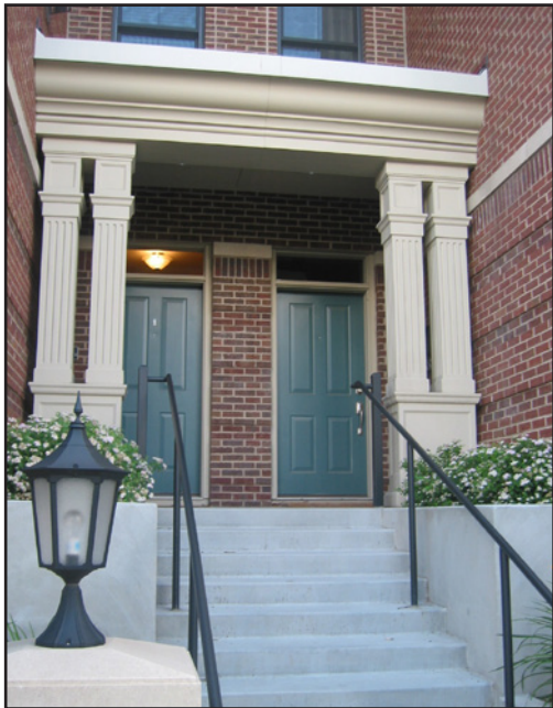
Recessed building entrances
