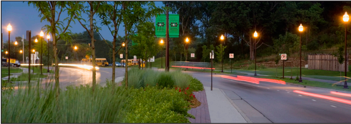
Enhance Beltline area's identity with attractive street lighting
