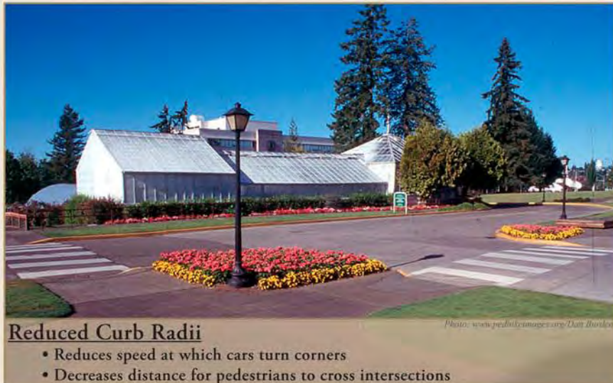
Reduced Curb Radii • Reduces speed at which cars turn corners • Decreases distance for pedestrians to cross intersections
