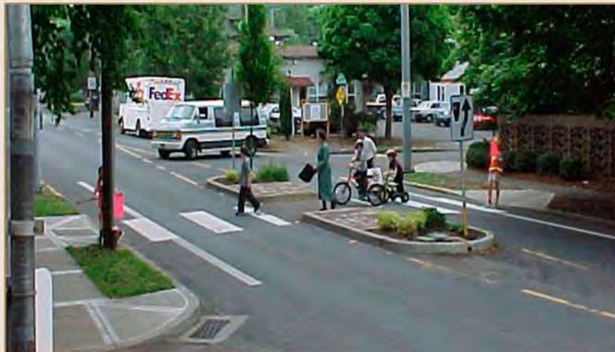
Pedestrian Refuge Island • Provides safer crossings for children, seniors & people with disabilities • Helps to reduce speed of vehicles
