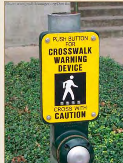
Accessible Pedestrian Signal • Audible indicator for pedestrian crossing
