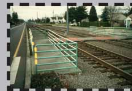
Example of a gating device which forces people to look both ways before crossing the railroad tracks
