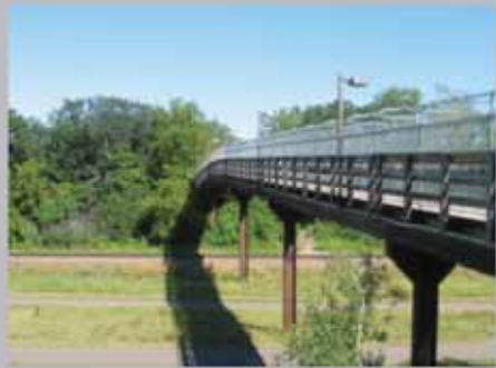
Existing pedestrian bridge over BNSF Railroads.
