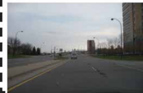
Xenia Ave, satisfactory for pedestrians, potentially unsafe for cyclists.
