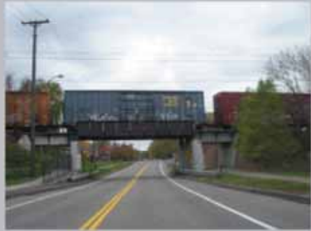
There are a few railroads that cross through the study area. These are barriers, but may be opportunities for trail sharing.
