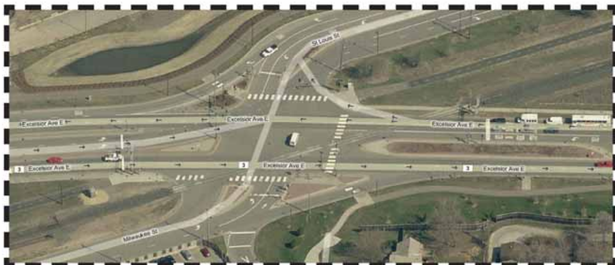
Precedent: At-grade crossing at the intersection of Excelsior Blvd and Milwaukee Street in Hopkins
