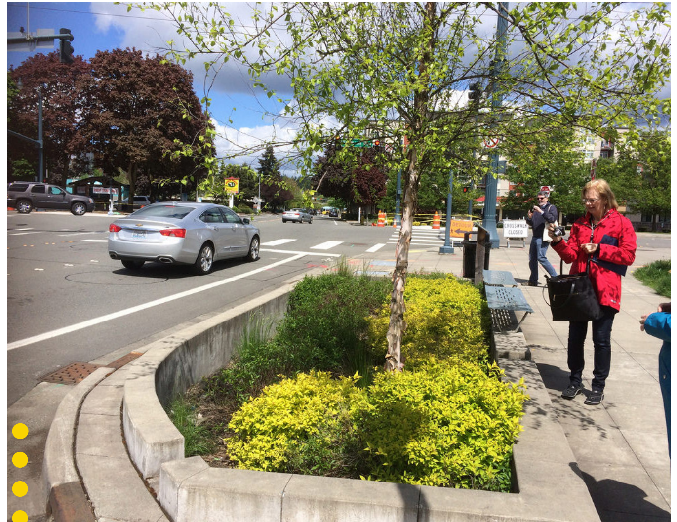
Public realm standards are designed to create a walkable, active streetscape but to also allow for flexibility and adherence to city standards.
