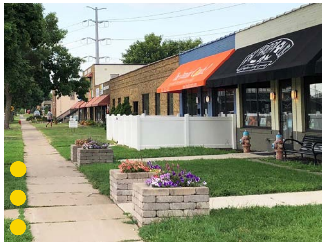
Historic Walker Lake is home to many businesses including these along Lake Street. Buildings are typically below two stories.
