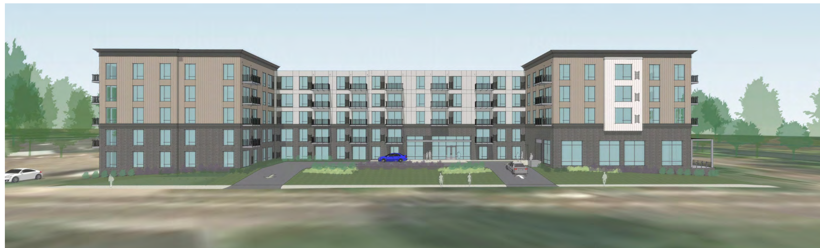
View of South Side
