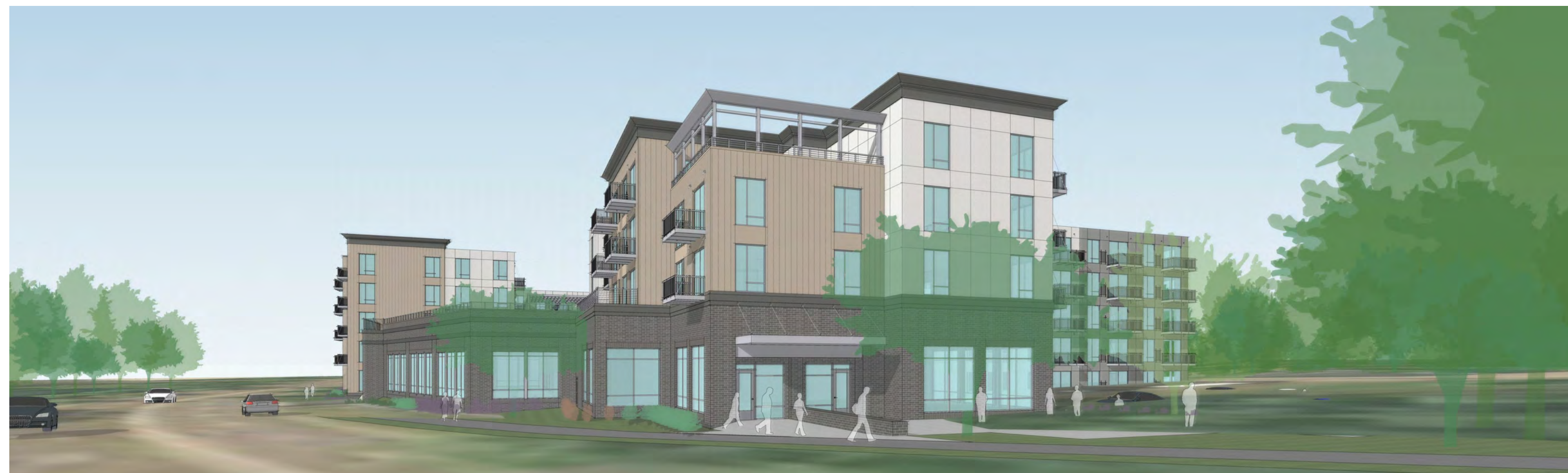
View of North Side
