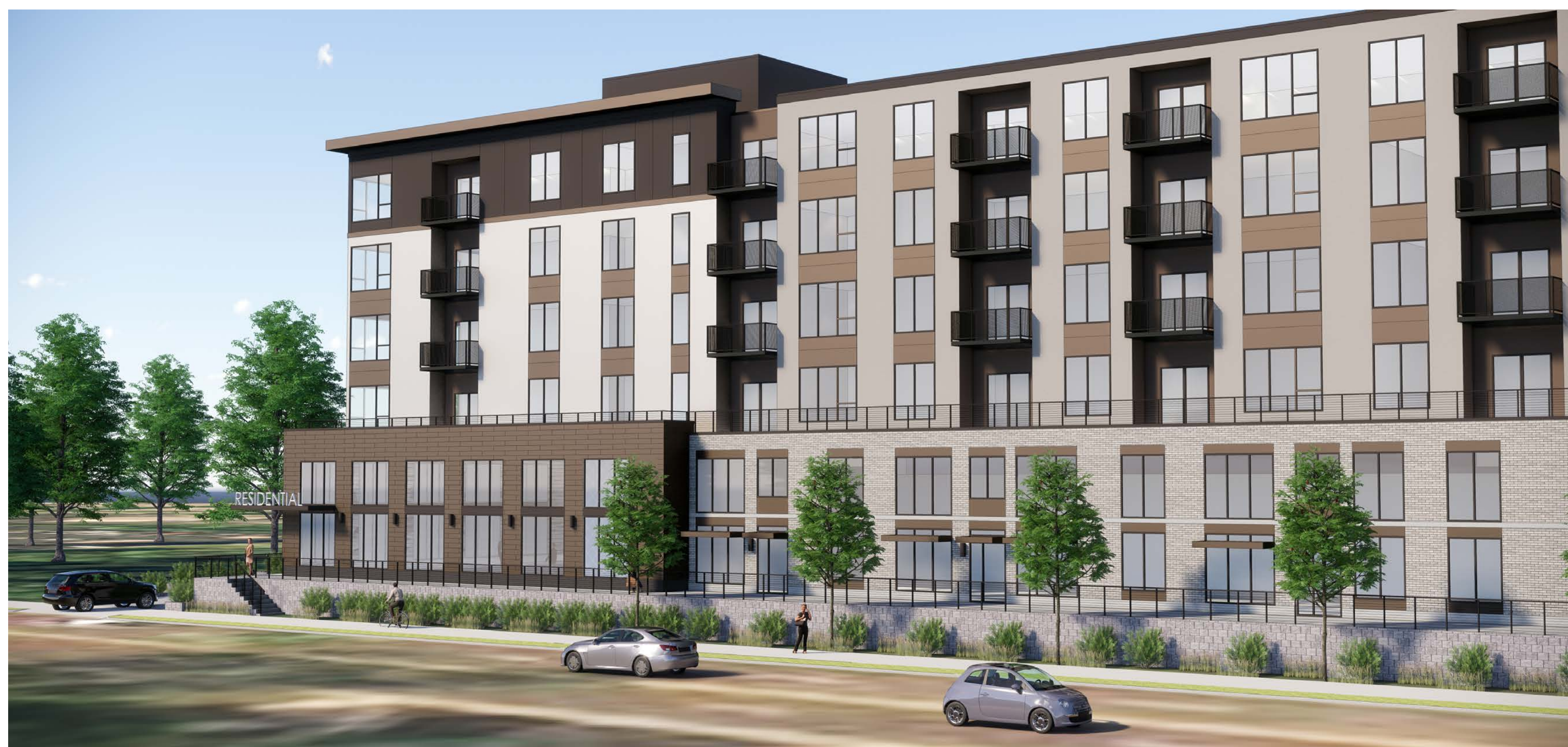
View from Beltline Boulevard Looking West
