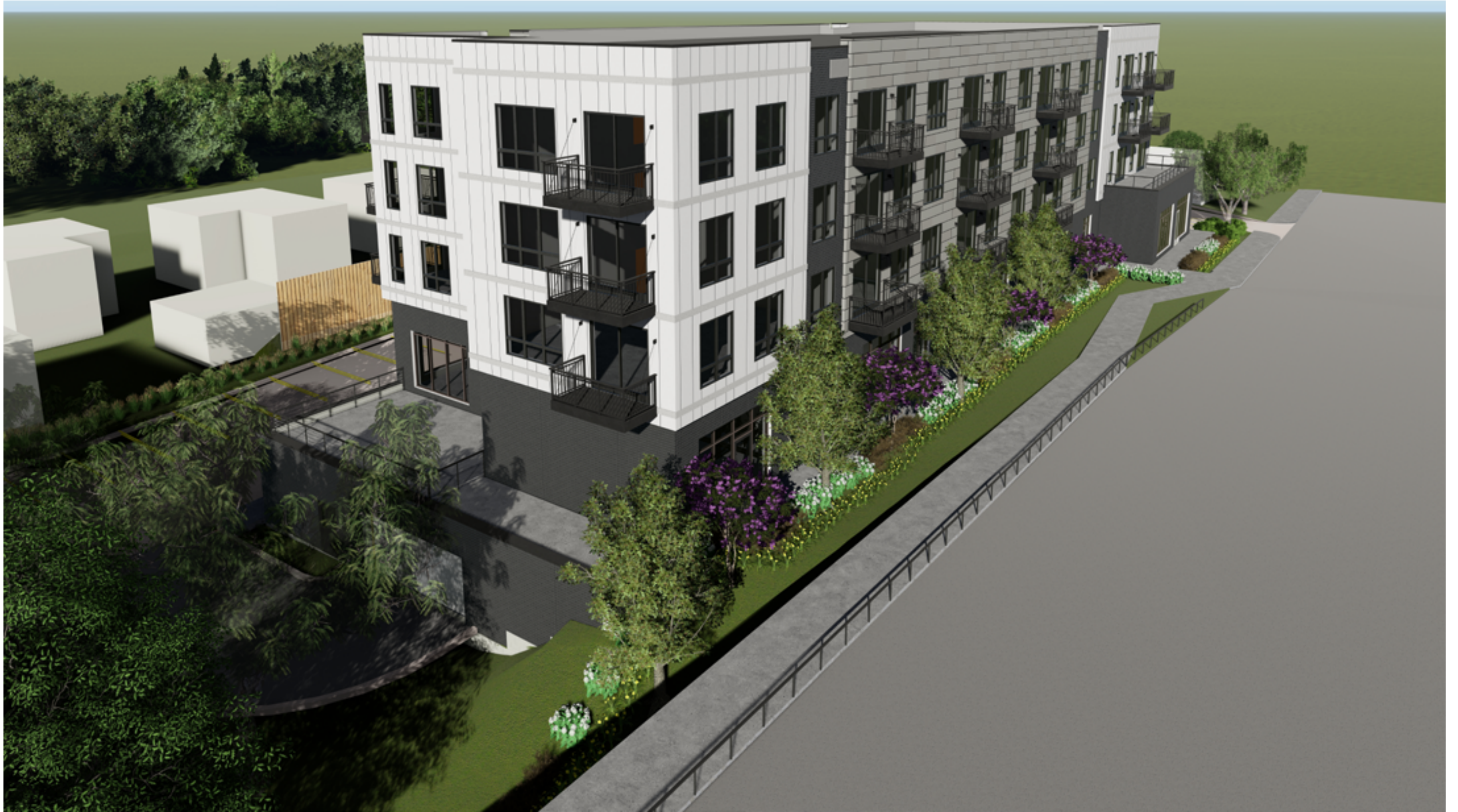
Aerial View looking Southeast
