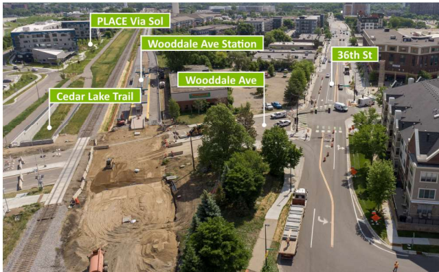
Wooddale Gateway area with 36th Street reconstruction, looking east
