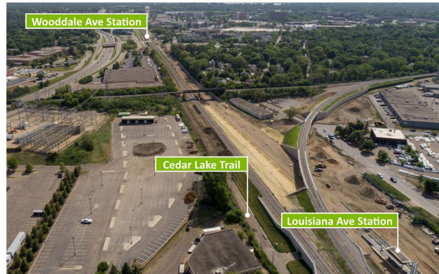
Louisiana Gateway area showing Metro Green Line LRT construction, looking east
