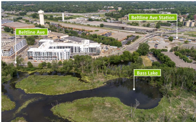
Beltline Gateway area, looking northwest
