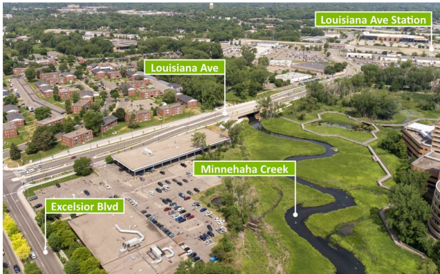
Excelsior Gateway area showing Minnehaha Creek and Louisiana Gateway area, looking north
