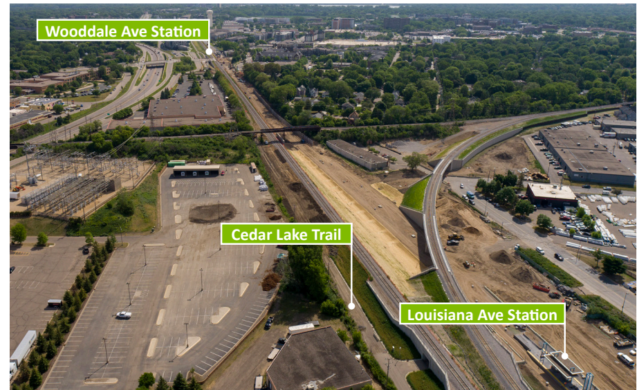
Louisiana Gateway area showing Metro Green Line LRT construction, looking east
