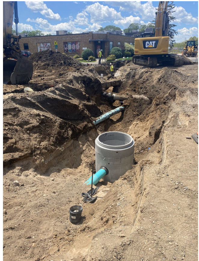
Underground utility construction
