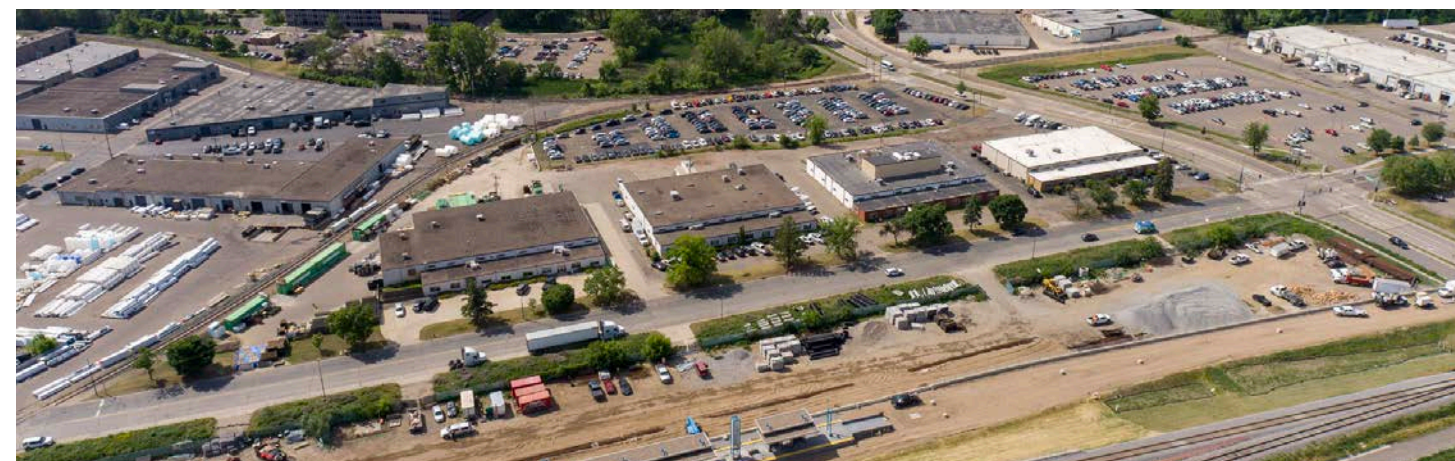
Existing Rail Spur
