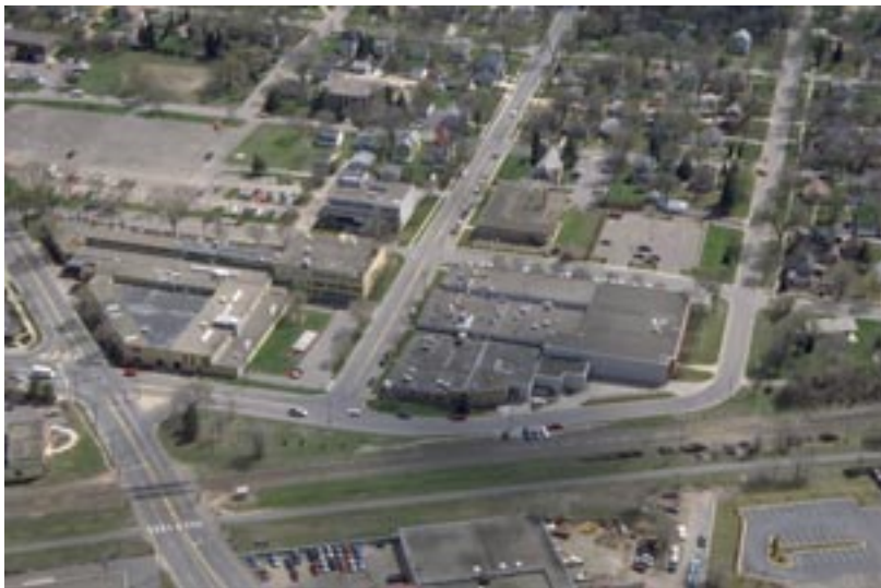
Quadion / Pechiney Looking South
